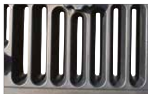
Slots in slatted floor allow natural cleaning of calves droppings.
